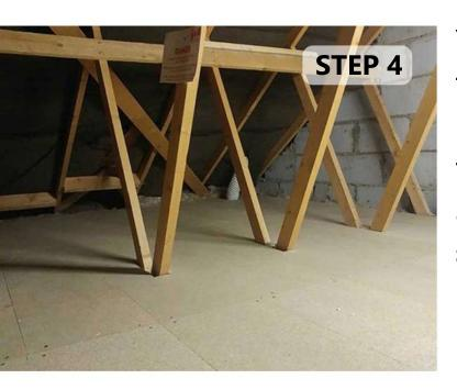
You can now board over with tongue and groove Loft Boards (1200mm x 325mm) or floor grade boards (600mm x 2400mm) to create a usable space for storage.
