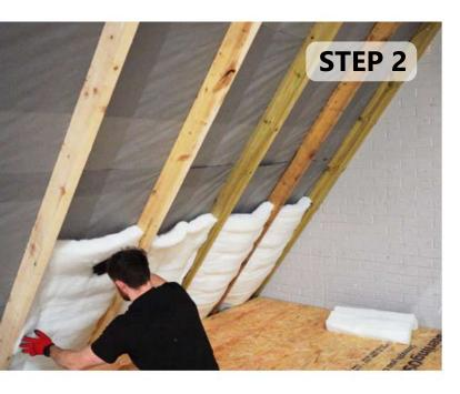
Install your EcoLoft Non-Itch between rafters, by rolling the material out between. You can cut the EcoLoft Non-Itch at the end of a run with our Multifoil Insulation Scissors to remove any excess, which can then be used to start your next run.
