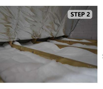
Roll out the EcoLoft Non-Itch and install between the floor joists. You can cut the EcoLoft Non-Itch at the end of a run with our Multifoil Insulation Scissors to remove any excess, which can then be used to start your next run.
