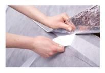
5. Fold the second roll back (100mm), remove the easy peel backing from the double sided tape and secure in place by applying pressure.
