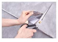
3. Breathe-R Ultra can be cut using a craft knife or sharp pair of scissors.
